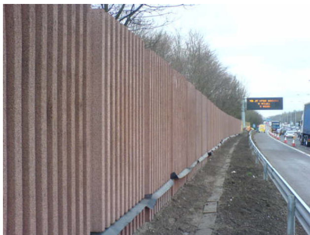
Figure 8: NOxer Barrier Section (Atkins, 2009).
